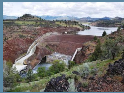
Iron Gate Dam and Powerhouse
