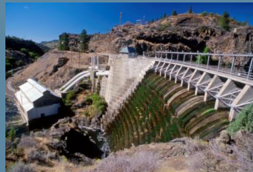
Copco No. 1 Dam and Powerhouse
