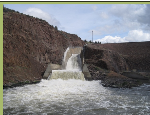
Iron Gate Dam Spillway
