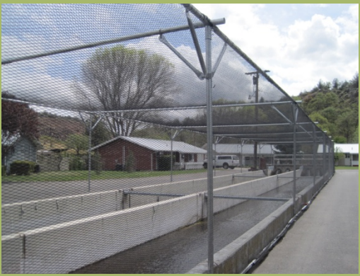
New Netting over Raceways at Iron Gate
