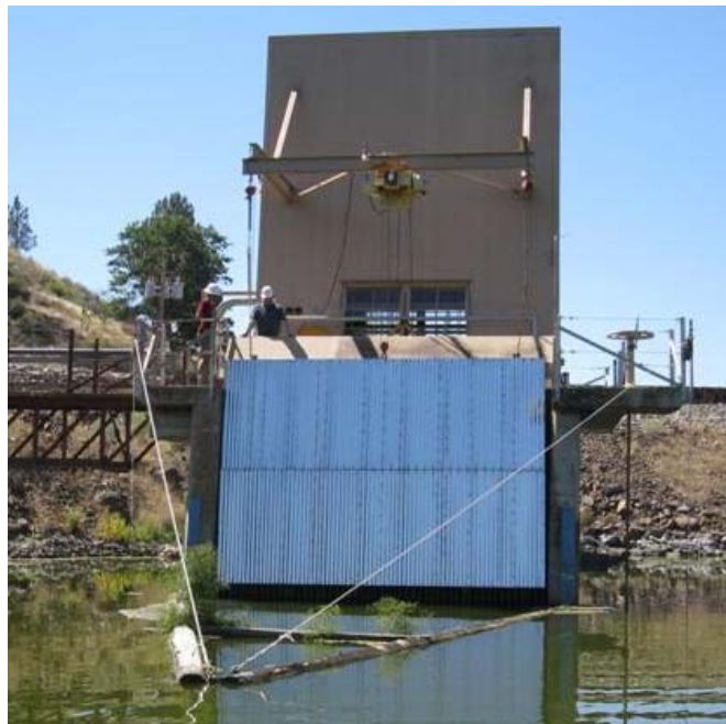
Figure 1. Iron Gate Intake Tower with cover installed, but not lowered.
