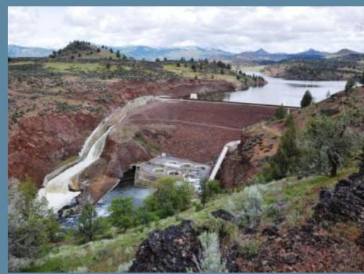
Iron Gate Dam and Powerhouse
