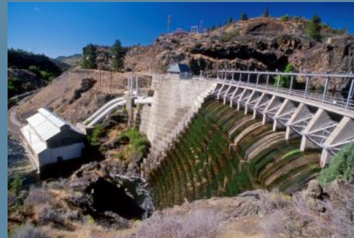
Copco No. 1 Dam
