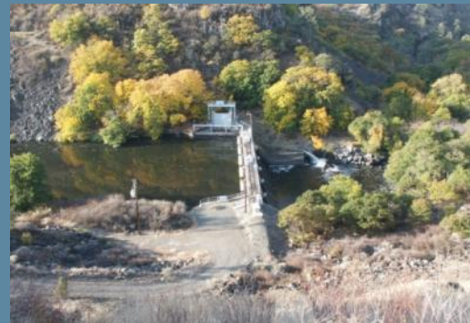
Copco No. 2 Dam
