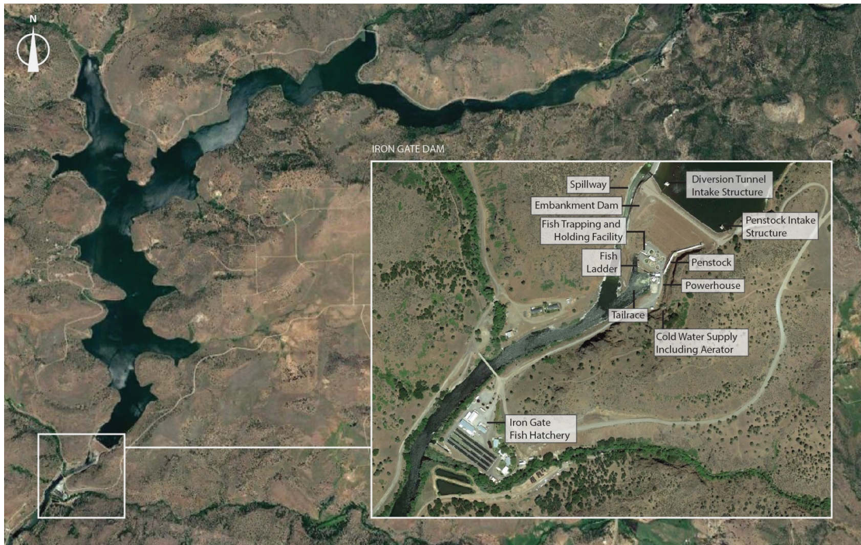
Figure 2.3-4. Iron Gate Dam and Associated Facilities.
