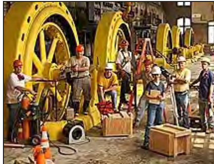
Preparations begin for rehabilitation of the Mechanicville Hydroelectric Project, Mechanicville, NY (photo Fourth Branch Associates)
