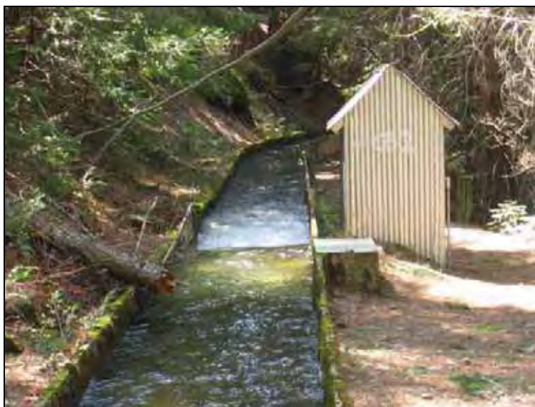
Feature 4: Gauging Station structure. Facing: Southwest (Photo acc. # 482-12-1-42)
