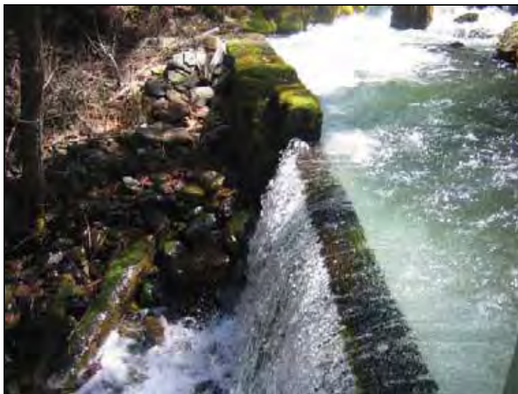
Feature 2: Diversion Dam. Facing: Northeast (Photo acc. # 482-12-1-39)
