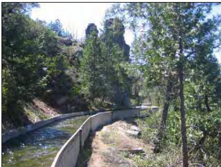
Feature 3: Concrete Canal. Facing: West (Photo acc. # 482-12-2-52)
