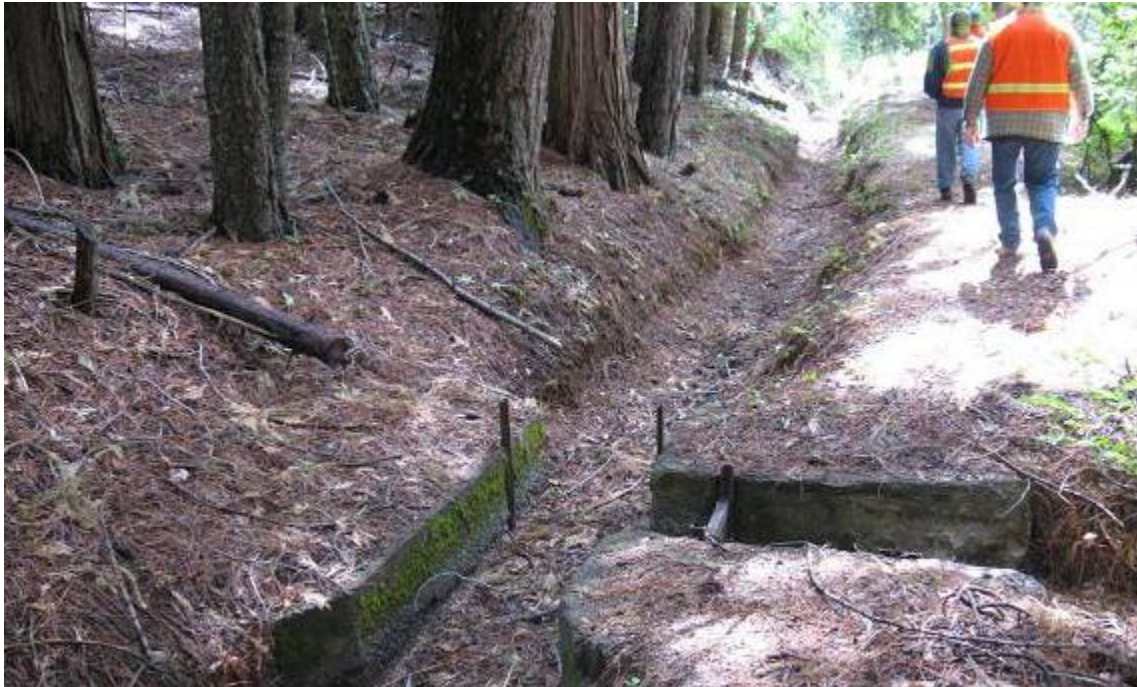
Photograph 2.2.2-1c South Canyon Creek – Canal and Spillway
