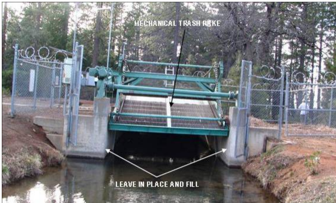
Photograph 2.2.5-1b Kilarc Forebay – Intake
