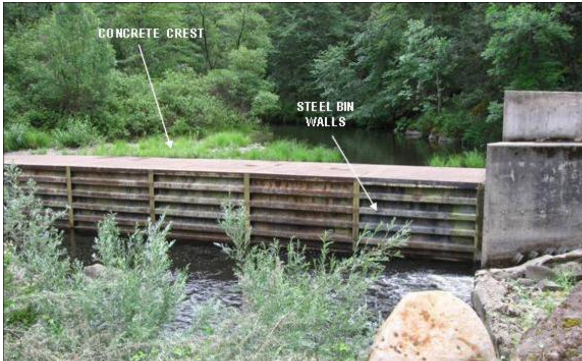
Photograph 2.3.3-1a South Cow Creek Diversion Dam
