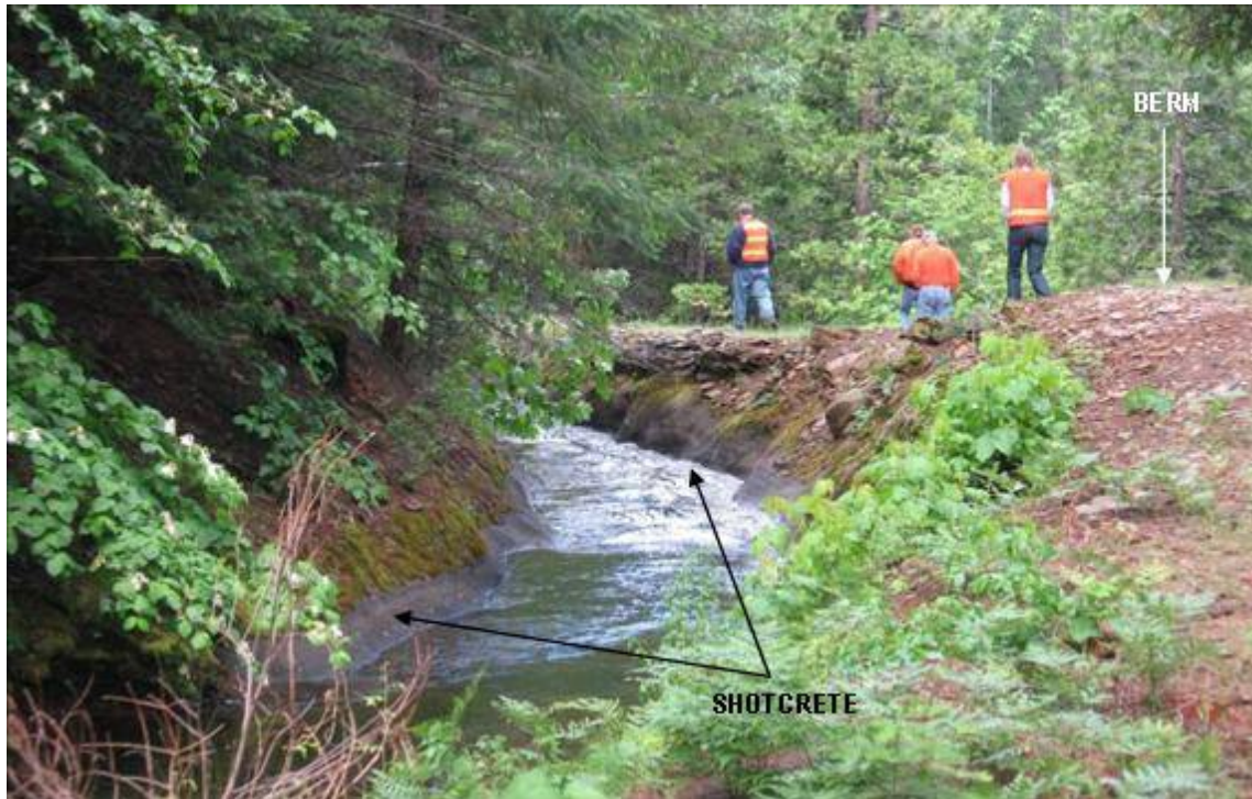
Photograph 2.2.4-1b Kilarc Main Canal – Shotcrete-Lined Section
