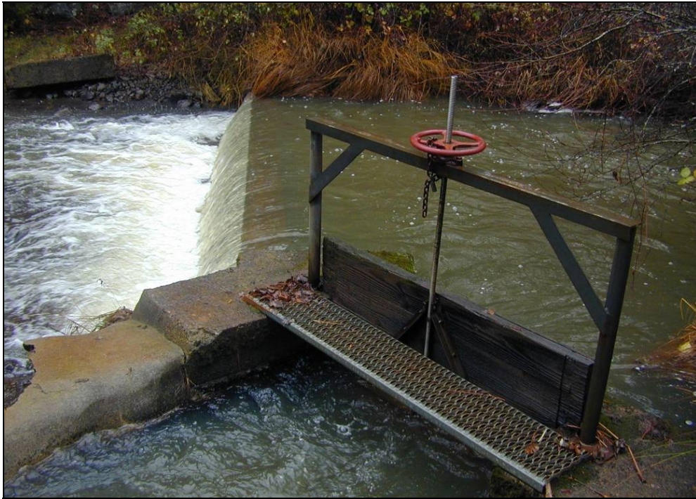
Photograph E.2.3-2. Mill Creek Diversion and Dam
