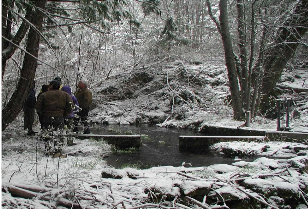
Photograph E.2.3-1. South Canyon Creek Dam and Diversion
