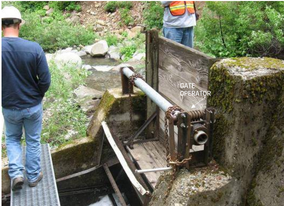
Photograph 2.2.3-1b Kilarc Main Canal Intake (View from Downstream Side of Gate)
