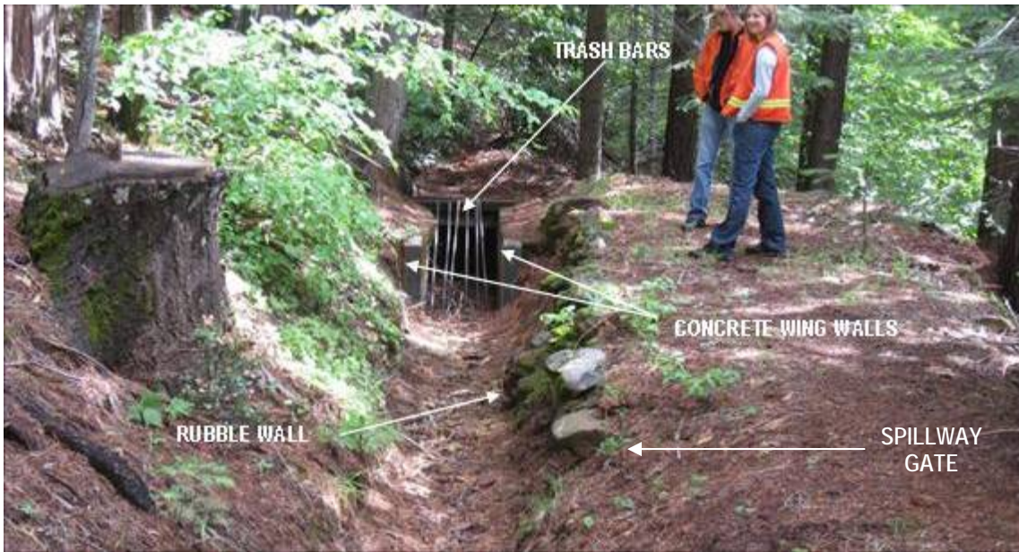
Photograph 2.2.2-1d South Canyon Creek – Canal Siphon Inlet
