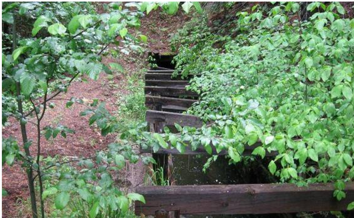
Photograph 2.2.4-1e Kilarc Main Canal – Tunnel
