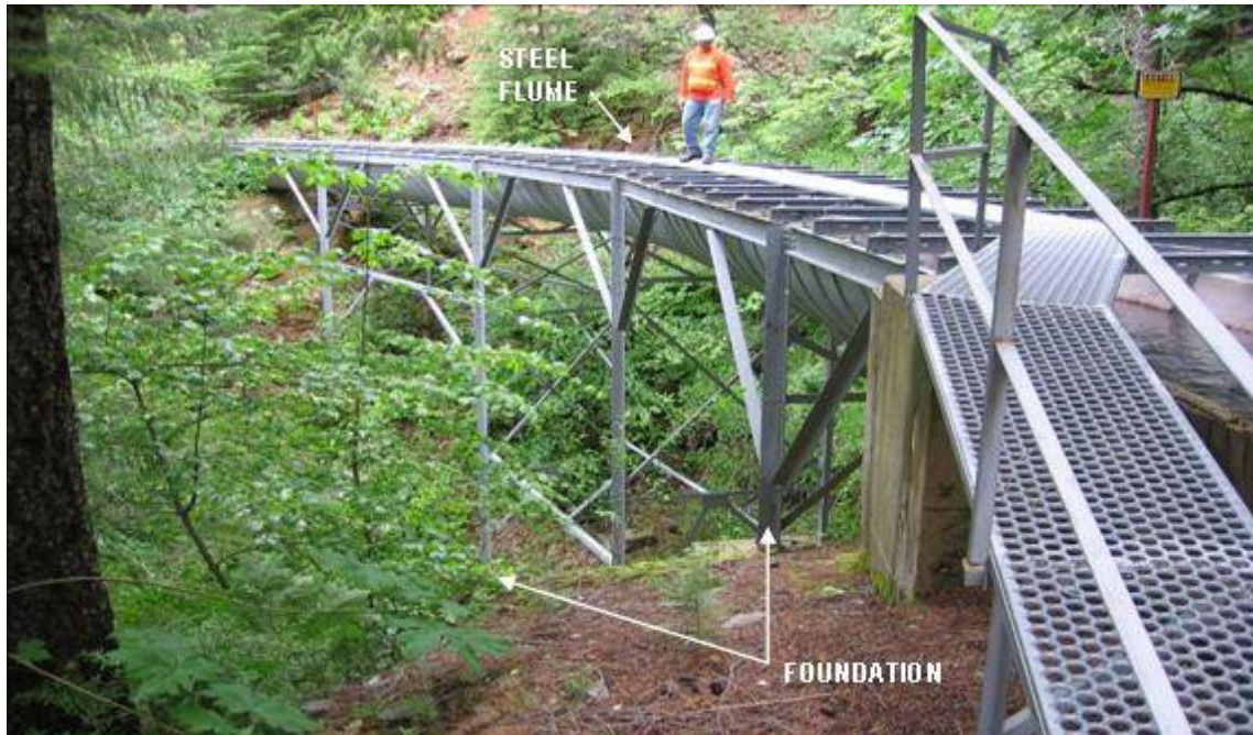
Photograph 2.2.4-1d Kilarc Main Canal – Steel Flume
