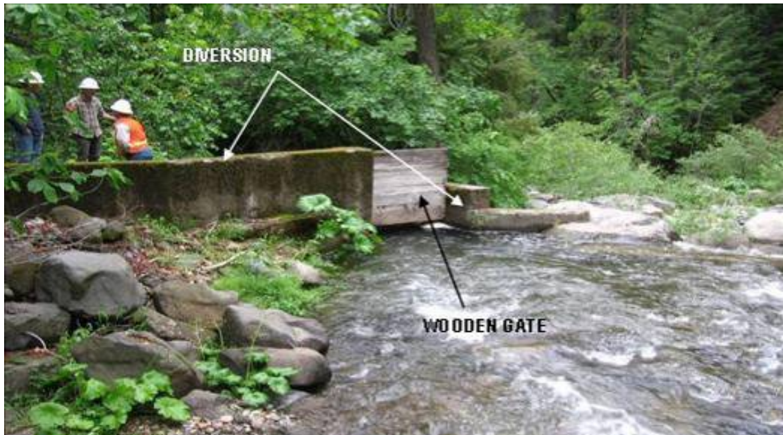
Photograph 2.2.3-1a Kilarc Diversion Dam (View from Upstream Side of Gate)
