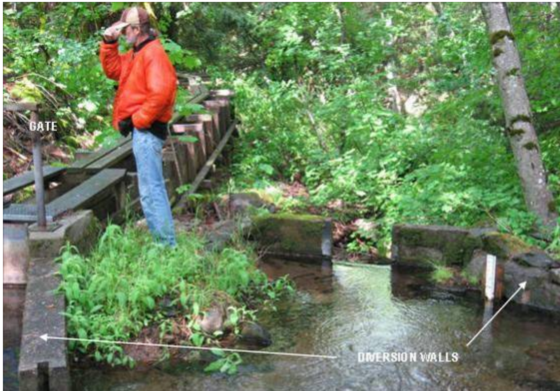
Photograph 2.2.2-1a South Canyon Creek – Diversion and Canal Inlet
