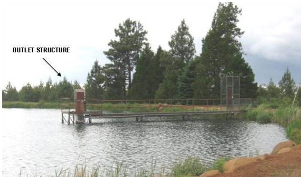
Photograph 2.2.5-1d Kilarc Forebay – Outlet Structure to Penstock
