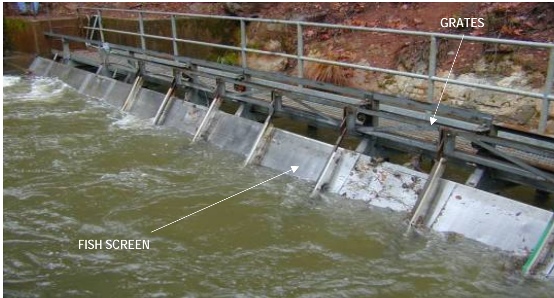
Photograph 2.3.3-1c South Cow Creek Diversion – Fish Screen Detail
