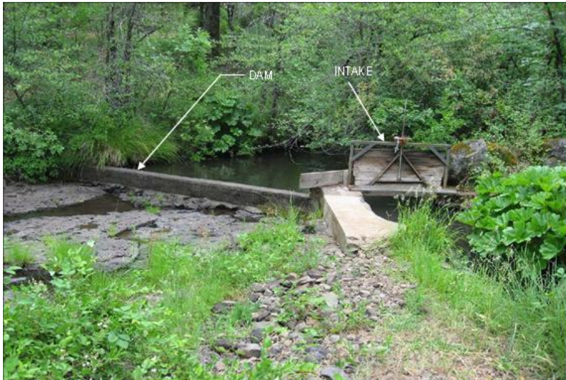
Photograph 2.3.1-1 Mill Creek Diversion – Dam and Canal Intake
