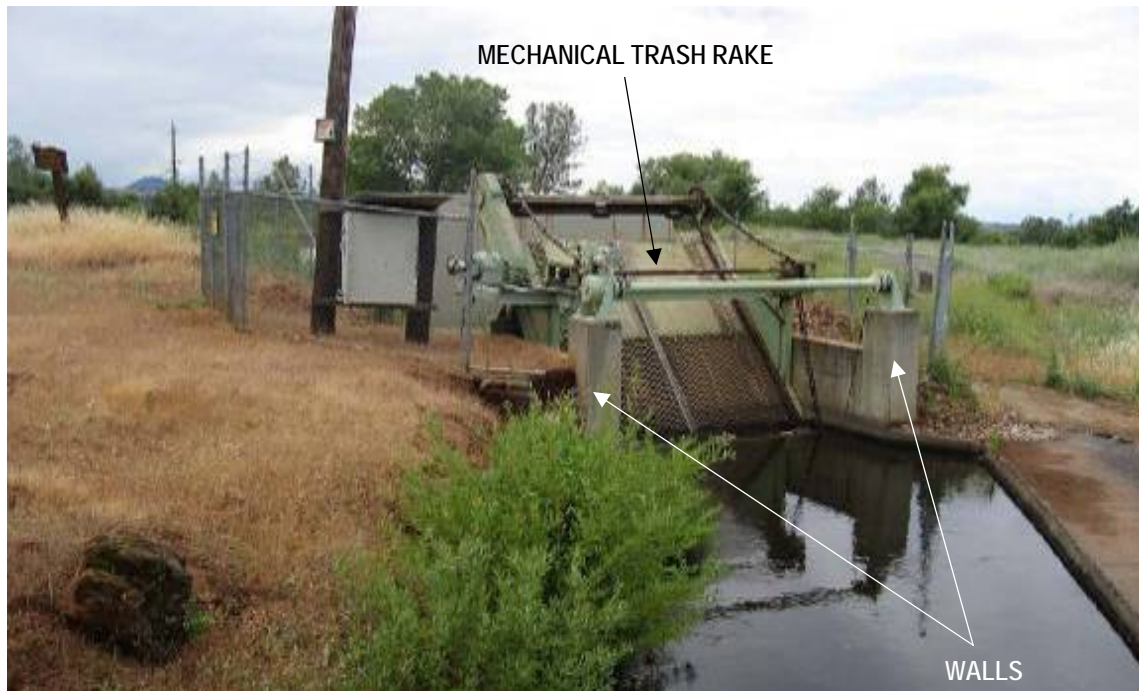
Photograph 2.3.5-1b Cow Creek Forebay – Intake
