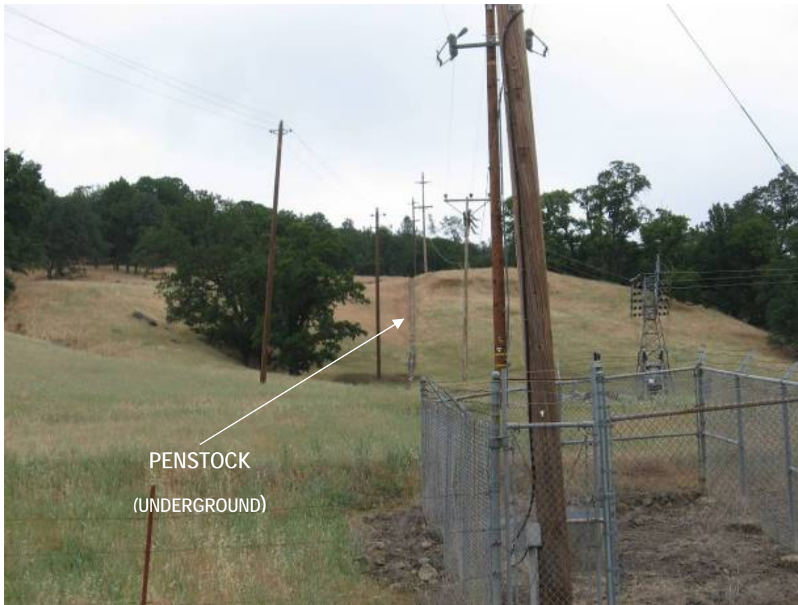
Photograph 2.3.7-1 Cow Creek – Penstock
