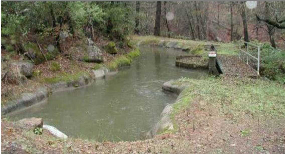
Photograph 2.3.4-1d South Cow Creek-Shotcrete Section
