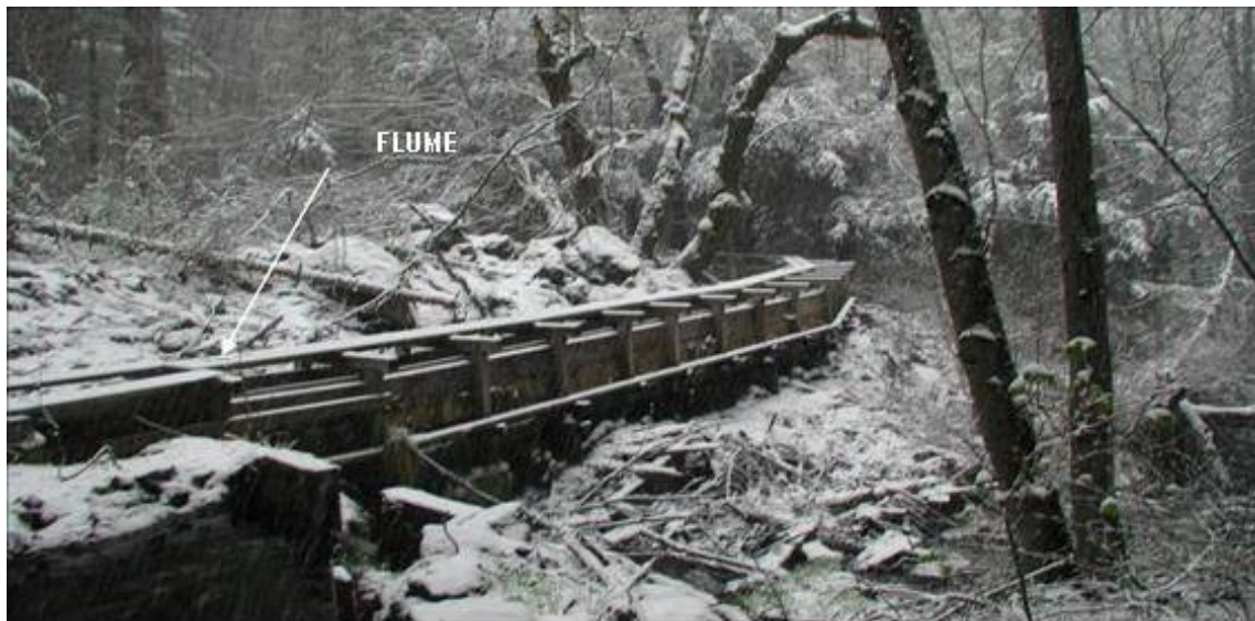
Photograph 2.2.2-1b South Canyon Creek – Canal Flumes
