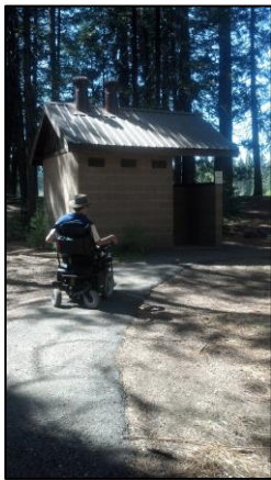
Figure 12: Restrooms, McCumber Lake
