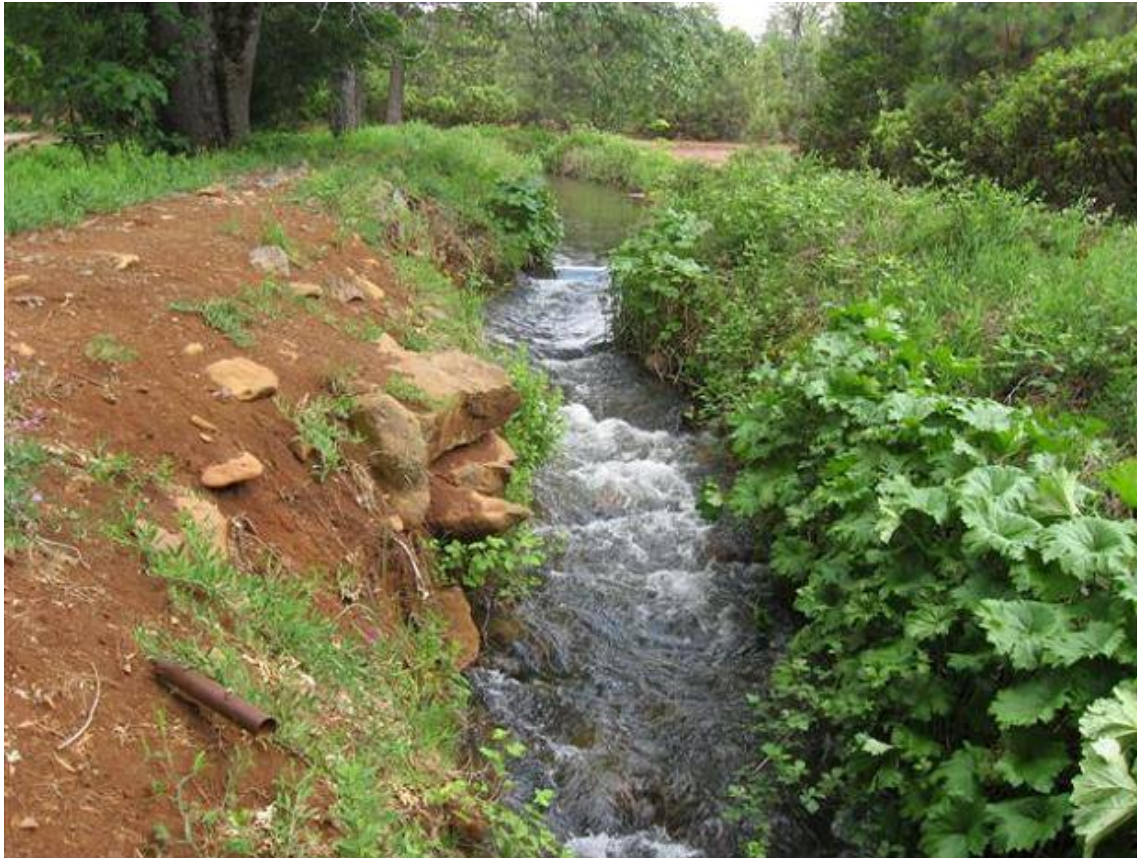
Photograph 2.2.4-1f Kilarc Main Canal – Earthen Section
