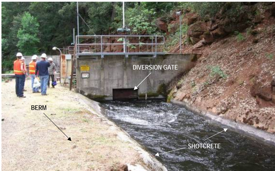
Photograph 2.3.4-1a South Cow Creek Canal
