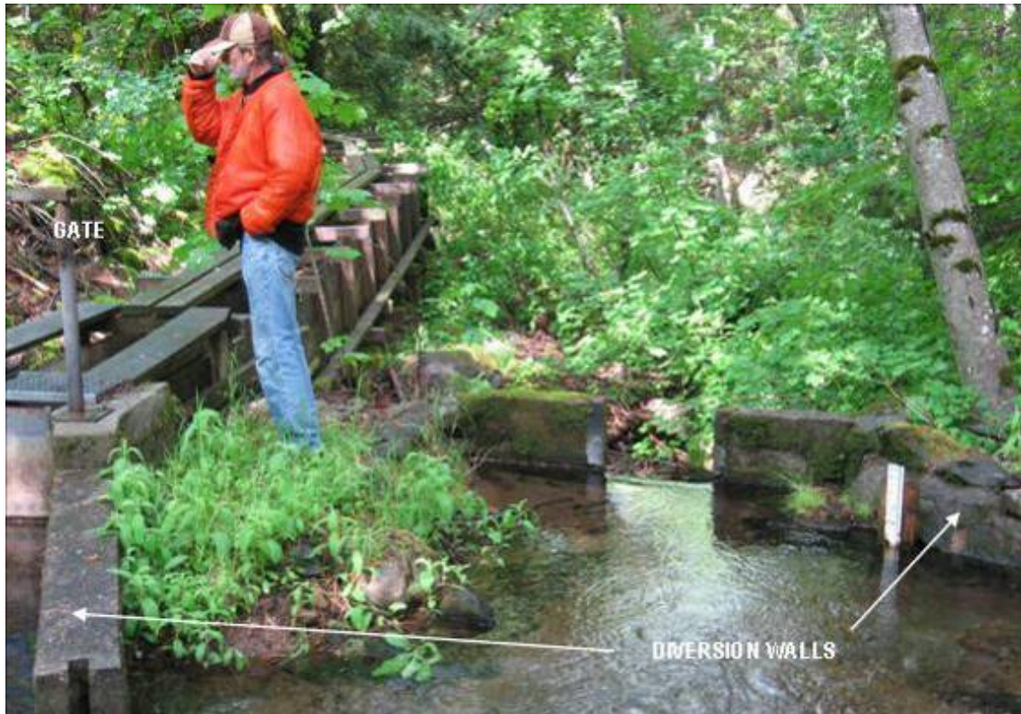
Photograph 2.2.2-1a South Canyon Creek – Diversion and Canal Inlet
