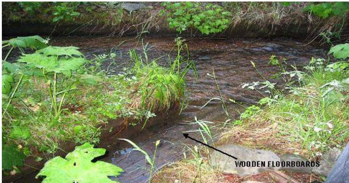
Photograph 2.2.1-1a North Canyon Creek – Diversion
