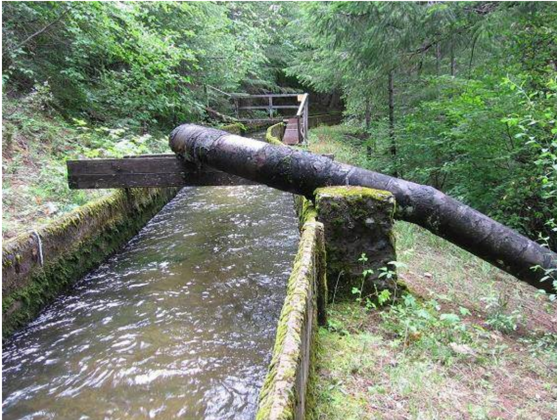
Photograph 2.2.2-1e South Canyon Creek – Canal Siphon Release To Kilarc Main Canal
