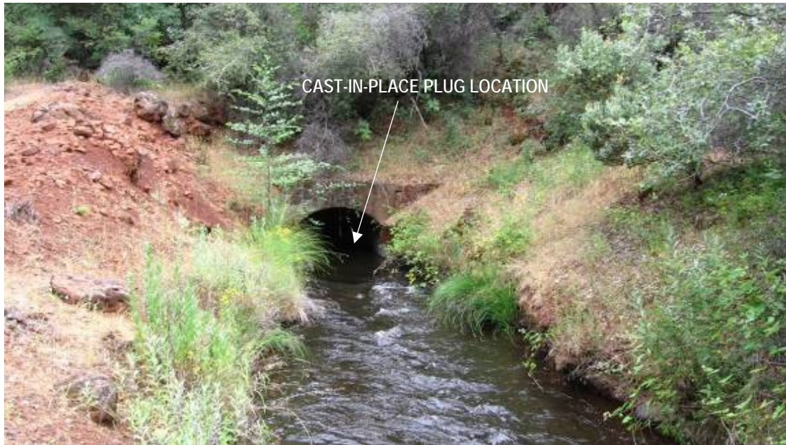
Photograph 2.3.4-1b South Cow Creek Tunnel
