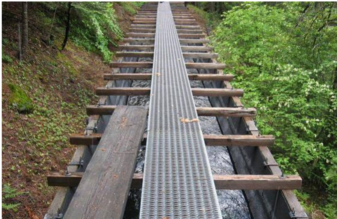
Photograph 2.2.4-1c Kilarc Main Canal – Wooden Flume
