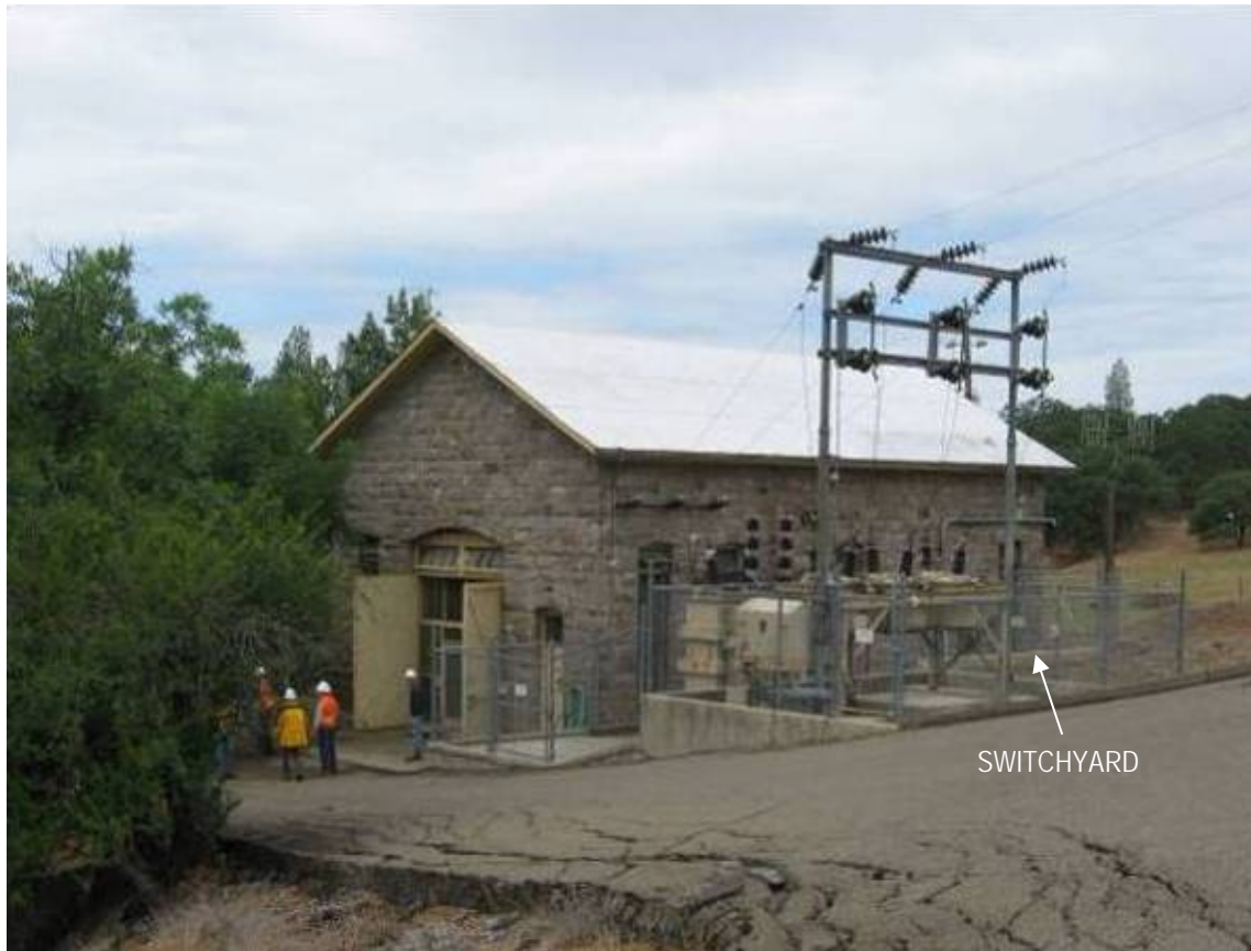
Photograph 2.3.8-1a Cow Creek – Switchyard and Powerhouse
