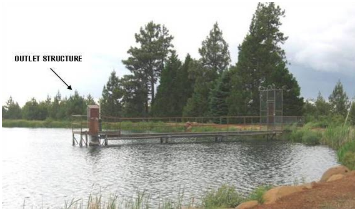
Photograph 2.2.5-1d Kilarc Forebay – Outlet Structure to Penstock
