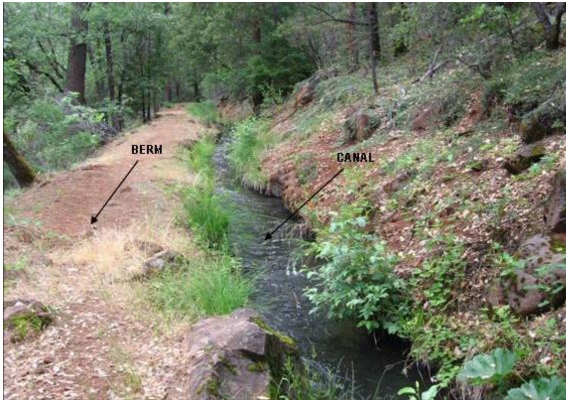
Photograph 2.3.2-1 South Cow Creek Canal
