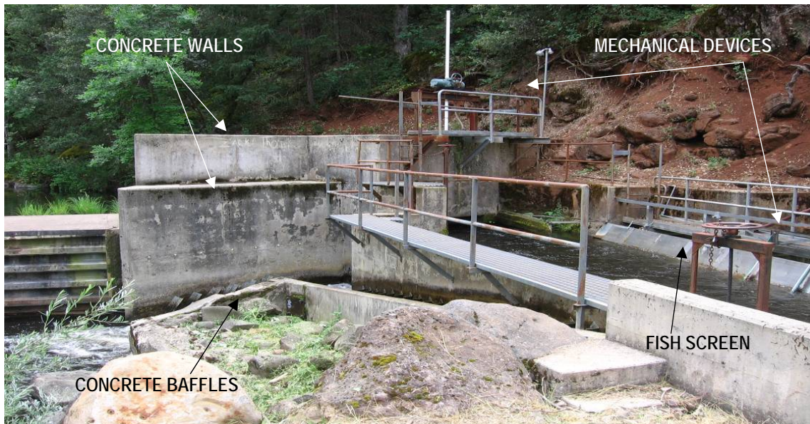
Photograph 2.3.3-1b South Cow Creek Diversion – Intake Structure and Fish Ladder
