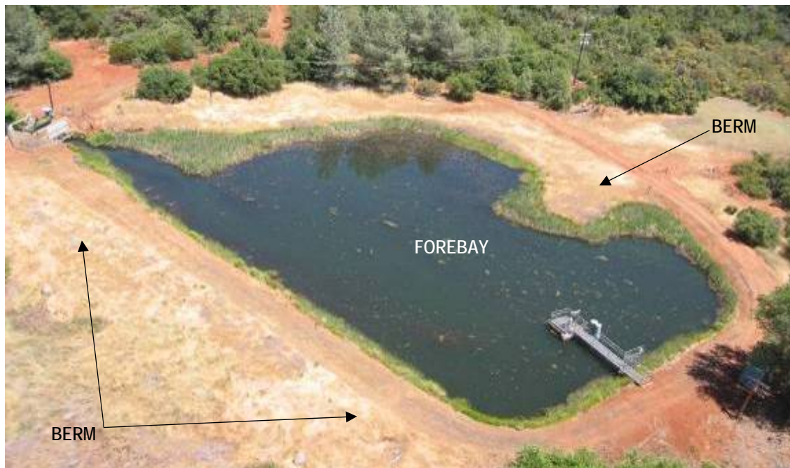
Photograph 2.3.5-1a Cow Creek Forebay and Outlet Structure
