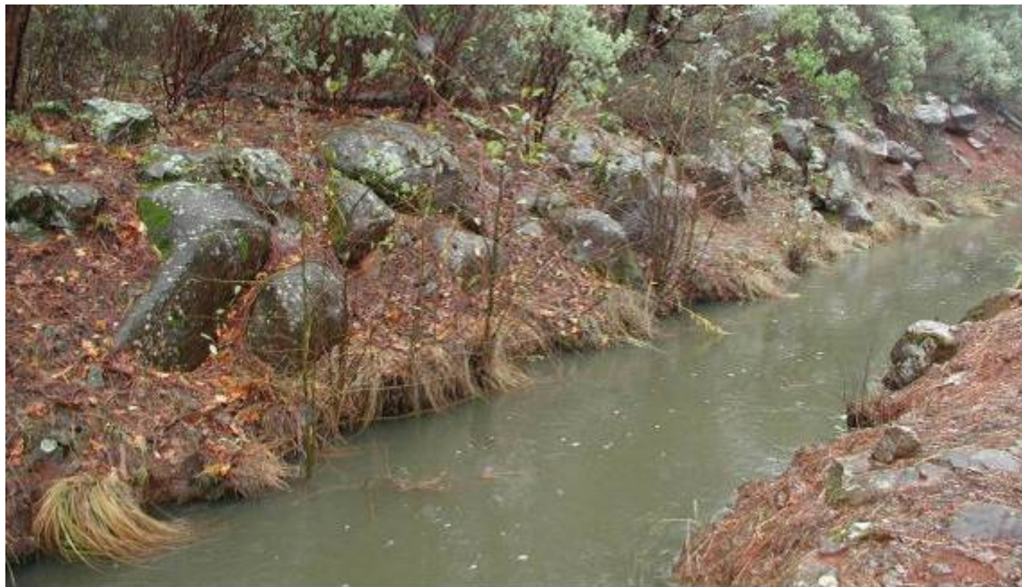
Photograph 2.3.4-1c South Cow Creek Canal-Earthen Section
