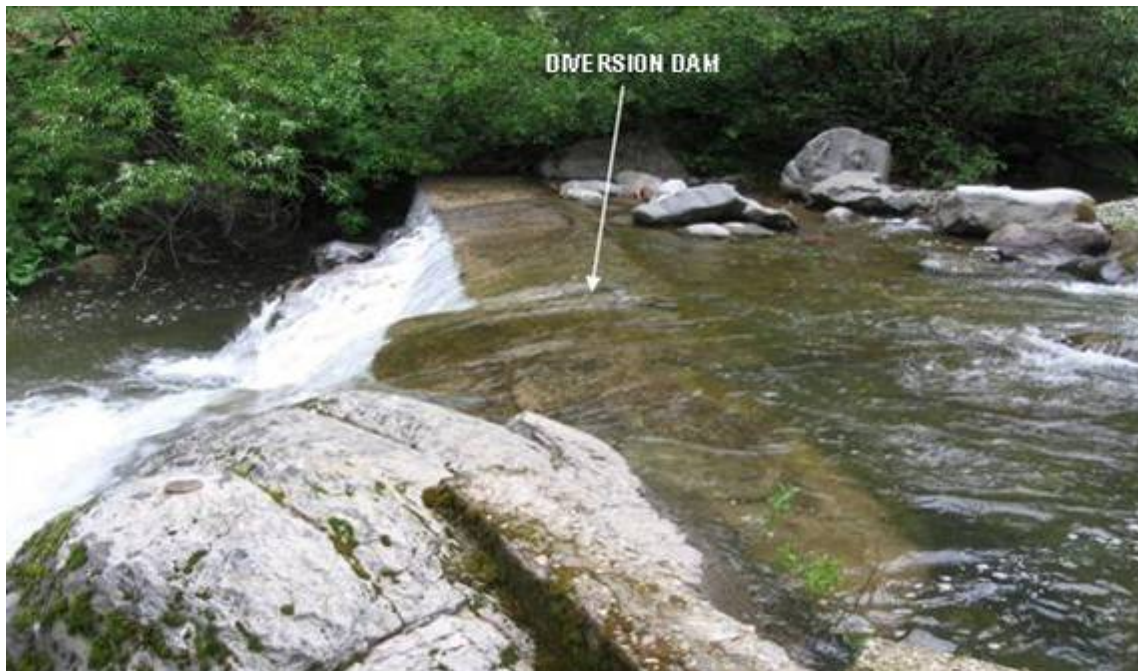
Photograph 2.2.3-1c Kilarc Main Canal – Diversion Dam
