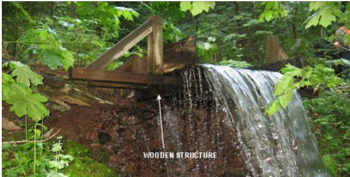
Photograph 2.2.1-1b North Canyon Creek – Wooden Structure to be Removed
