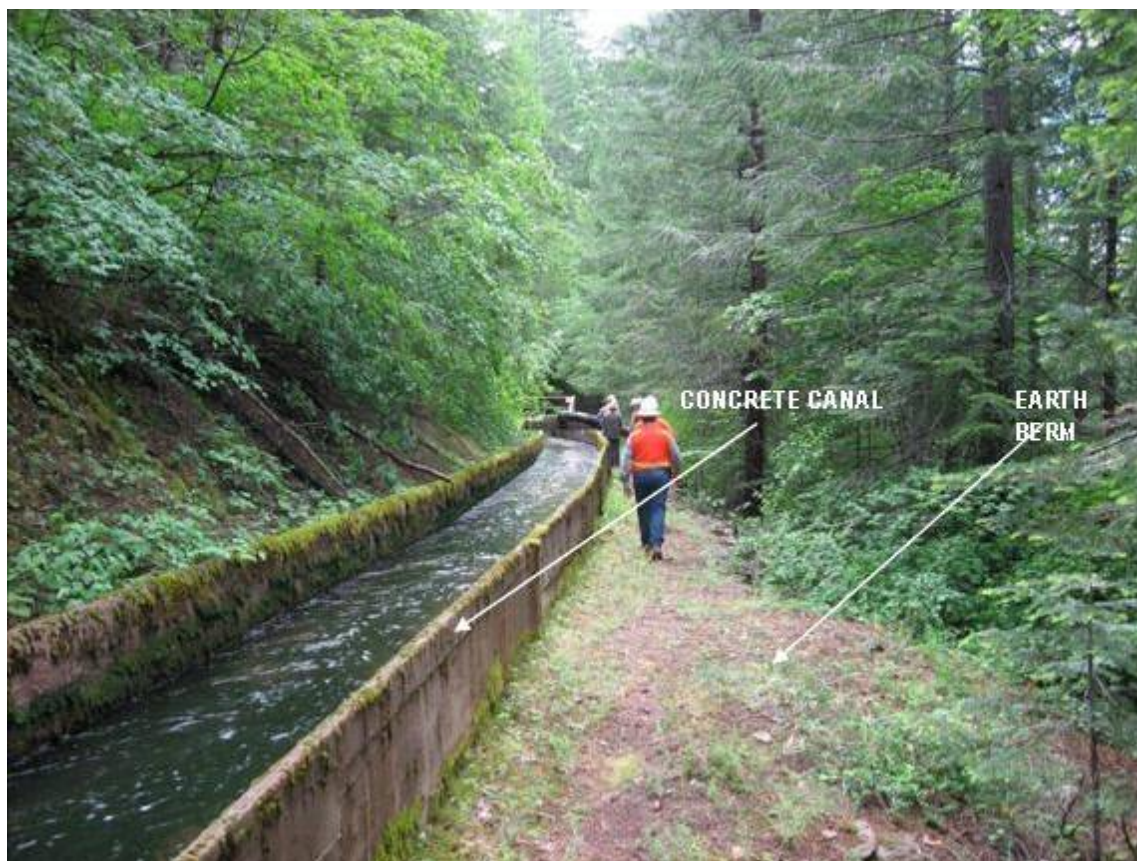
Photograph 2.2.4-1a Kilarc Main Canal – Concrete Section
