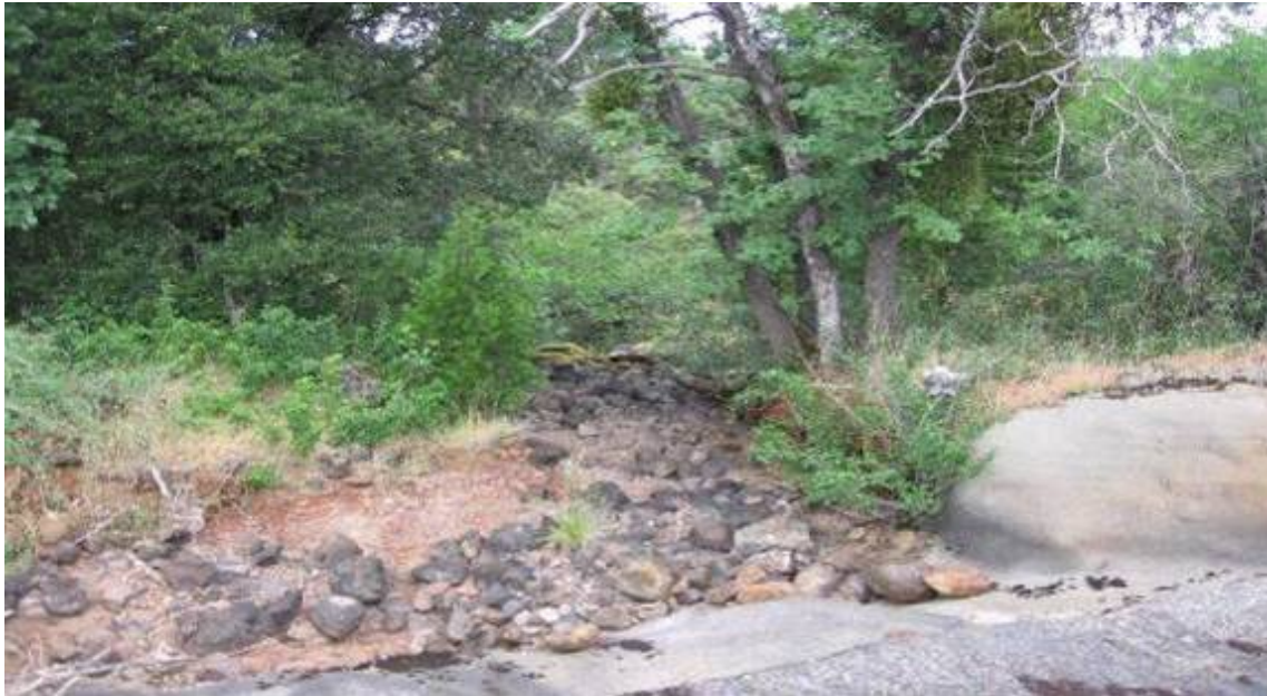
Photograph 2.3.5-1d Cow Creek Forebay – Spill Outlet
