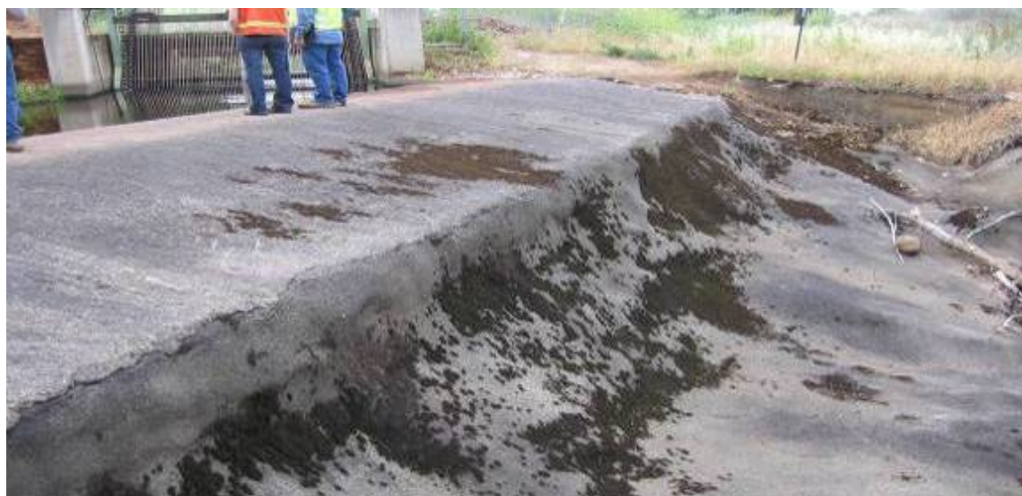
Photograph 2.3.5-1c Cow Creek Forebay – Spill Channel
