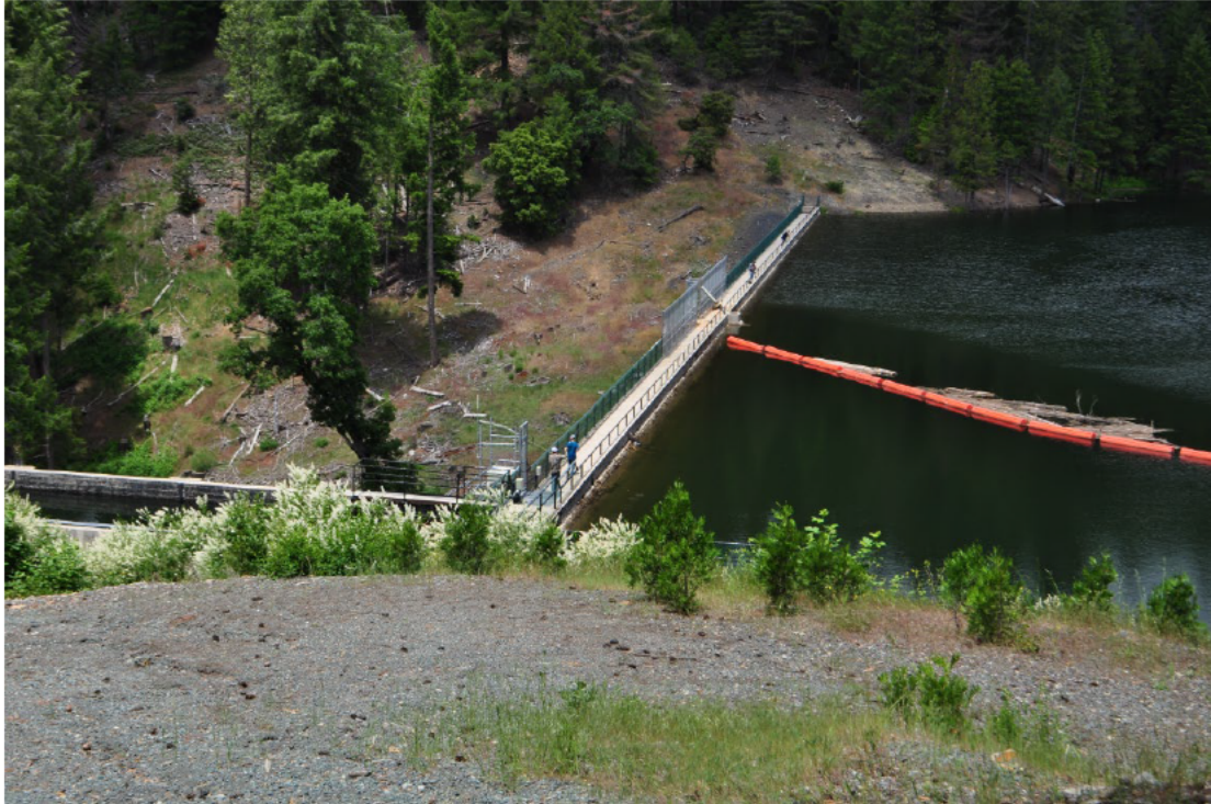
Key View 7. View from Spur 7 looking northwest toward the existing spillway structure, dam, reservoir, and location of the proposed spillway.
