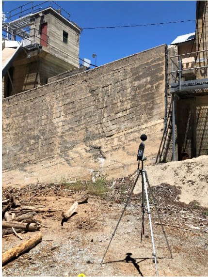
ST-1 Looking North
