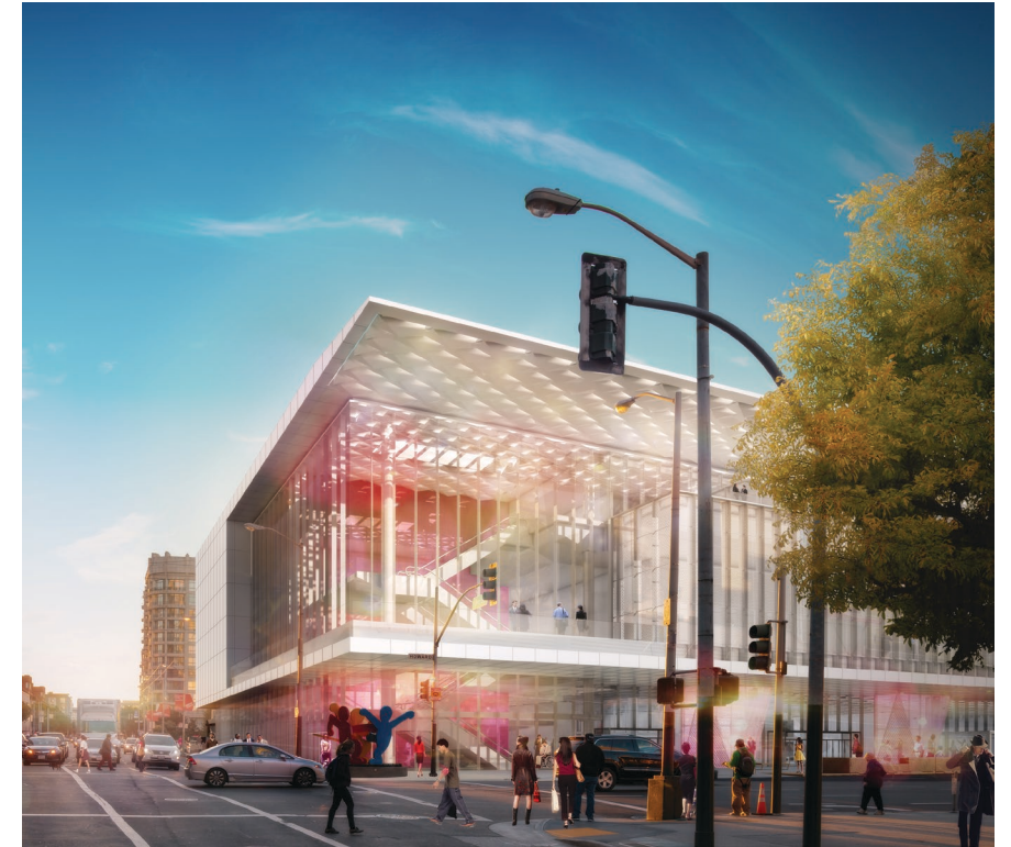
Moscone Center in SF captures, treats, and reuses 46 AF of rainwater, drainage, and steam condensate annually.
